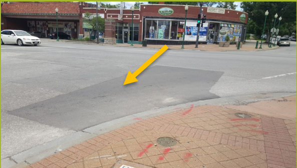
EXAMPLES OF RECENT TEMPORARY POTHOLE REPAIRS ALONG THE AVENUE
