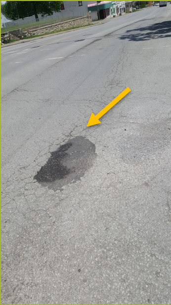
EXAMPLES OF RECENT TEMPORARY POTHOLE REPAIRS ALONG THE AVENUE
