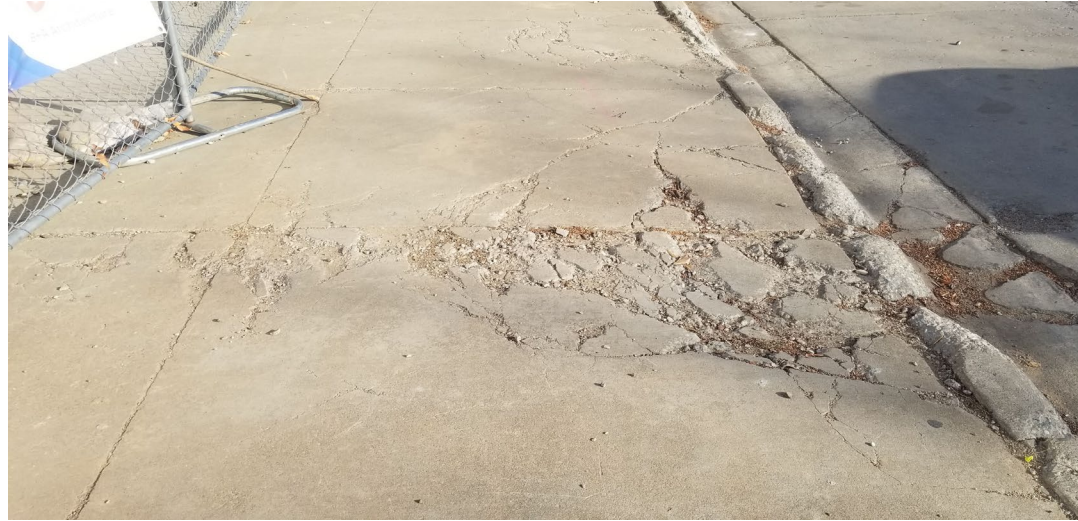
Broken, damaged and worn sidewalks
