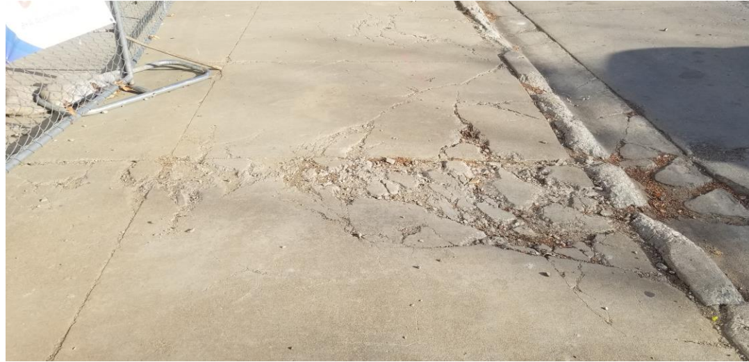
Broken, damaged and worn sidewalks
