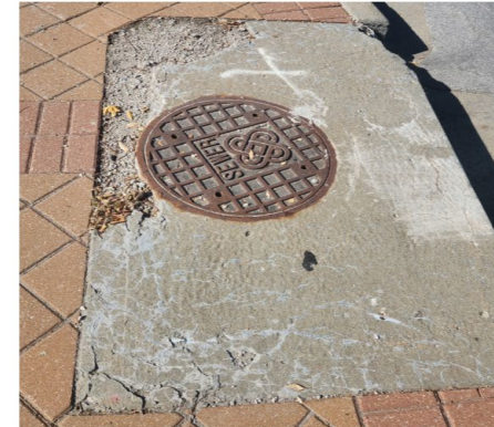
Replace drain inlets
