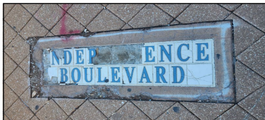
PIAC PROJECT OBJECTIVE—REPLACE MISSING AND DAMAGED TILES, MORTAR AS NEEDED
