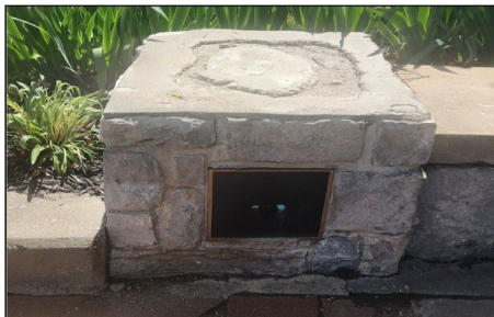
PIAC PROJECT OBJECTIVE—REPLACE MISSING CONCRETE TOPS, MORTAR AS NEEDED
