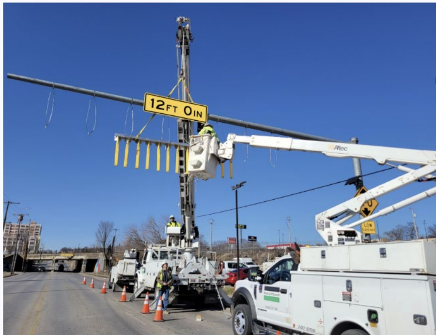
Photo Courtesy of Michael Bushnell | Crews with Black & McDonald re-hanging the recovered piece of the warning curtain system.
